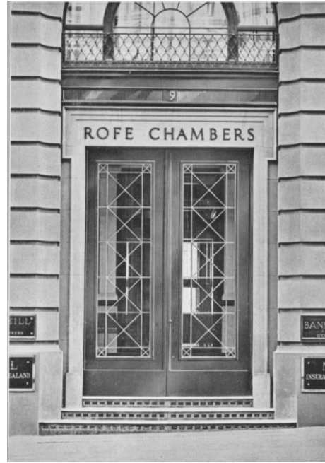
7 Bronze encased entrance doors to Rofe Chambers, Sydney Source: 40 years of Wunderlich
