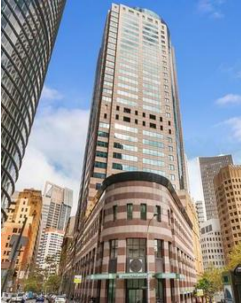
The Wintergarden, 1-15 O'Connell Street
